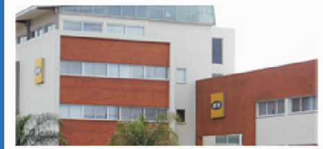
MTN Building, South Africa
